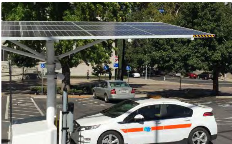
Solar powered EV charging station at Caltrans Headquarters
