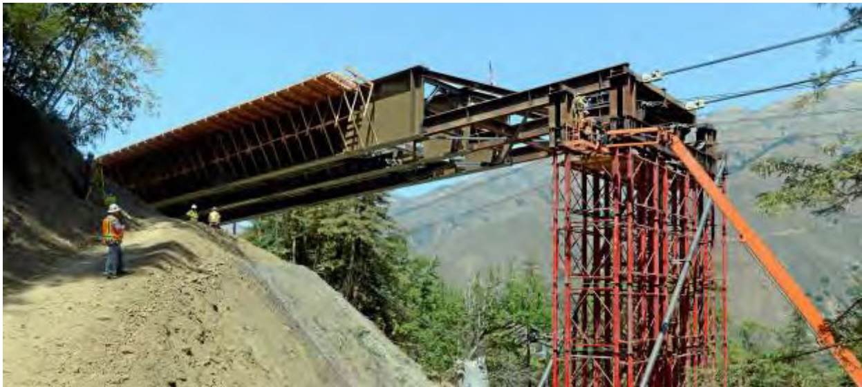
Pfeiffer Canyon Bridge Launch
