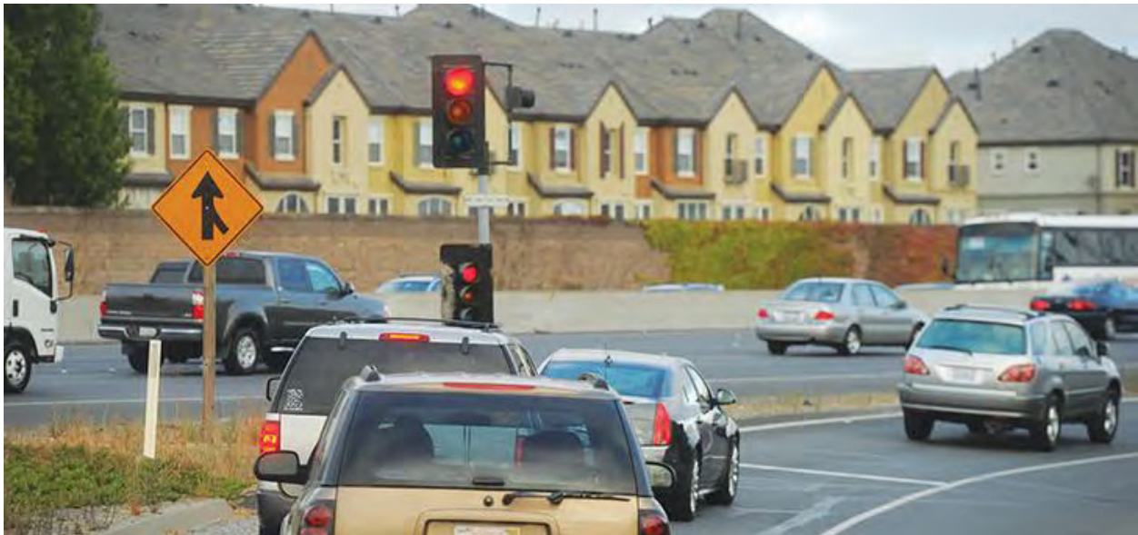
Bay Area Ramp Meter (source: MTC)
