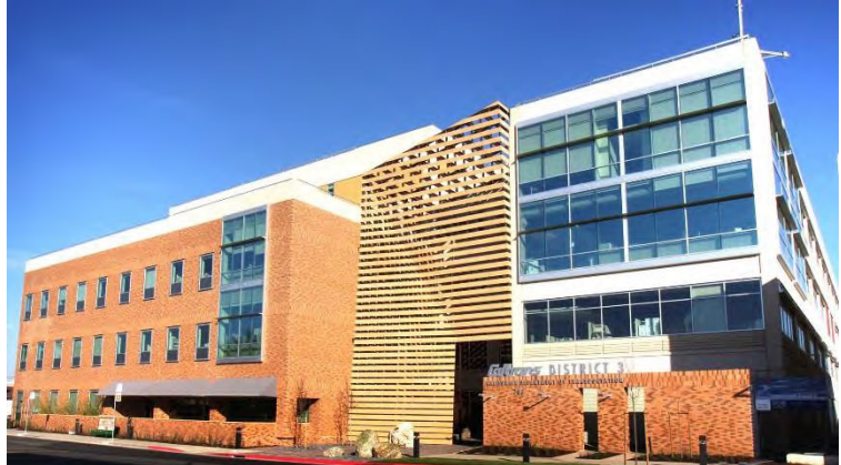
District 3 Headquarters, Marysville, CA
