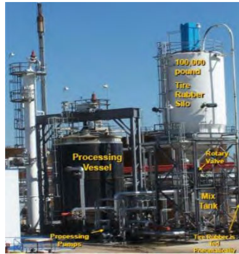
Terminal Blending Process for Rubberized Asphalt
