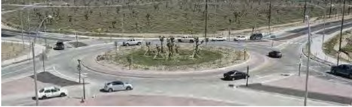
Roundabout on Route 138 in Palmdale
